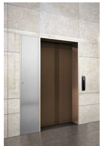
Entrance with control panel
